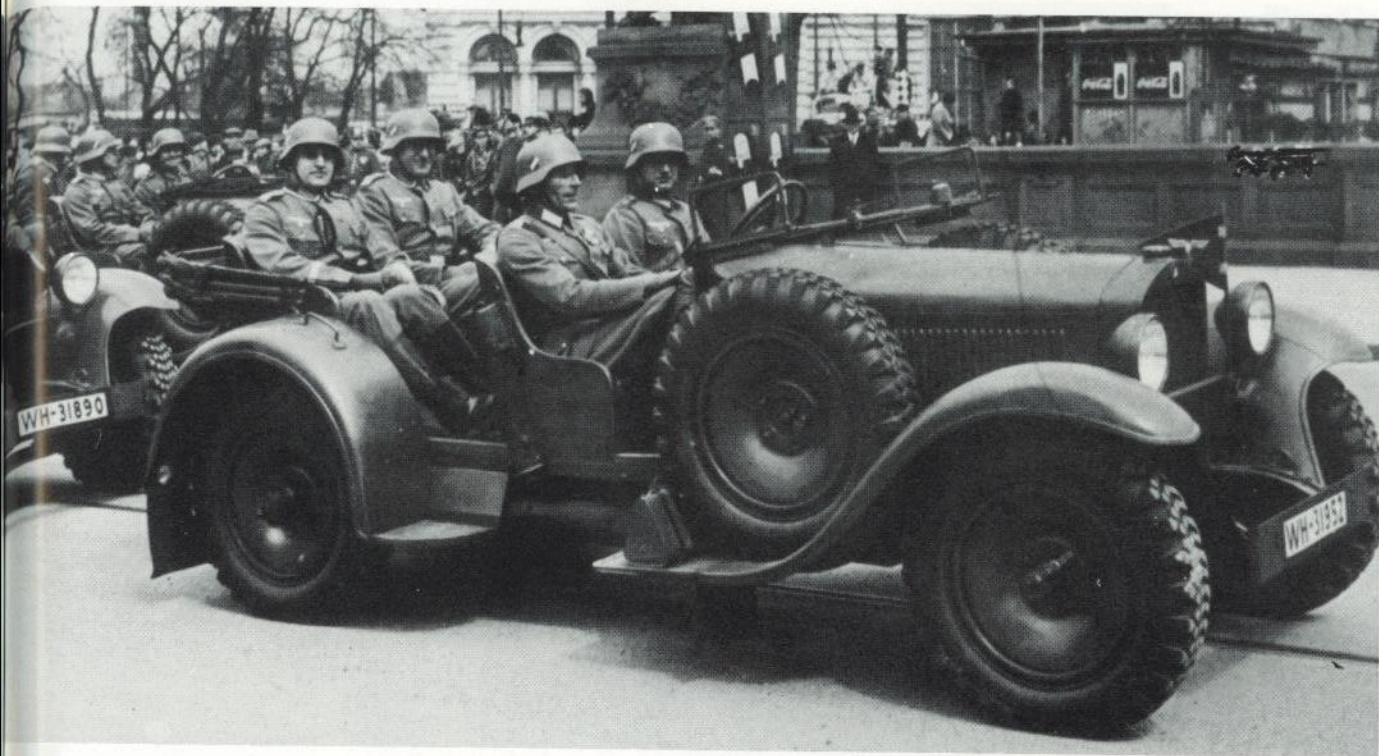
Left: The best-looking of all “bucket cars” was probably the Mercedes-Benz Stuttgart 260. It was built from 1929 to 1935 and had a straight 6-cylinder motor with 2.6- liter displacement and 50- HP performance. The picture shows the Fla Instructional Company (Captain von der Mosel) in the 1936 Leader’s Parade in Berlin.
