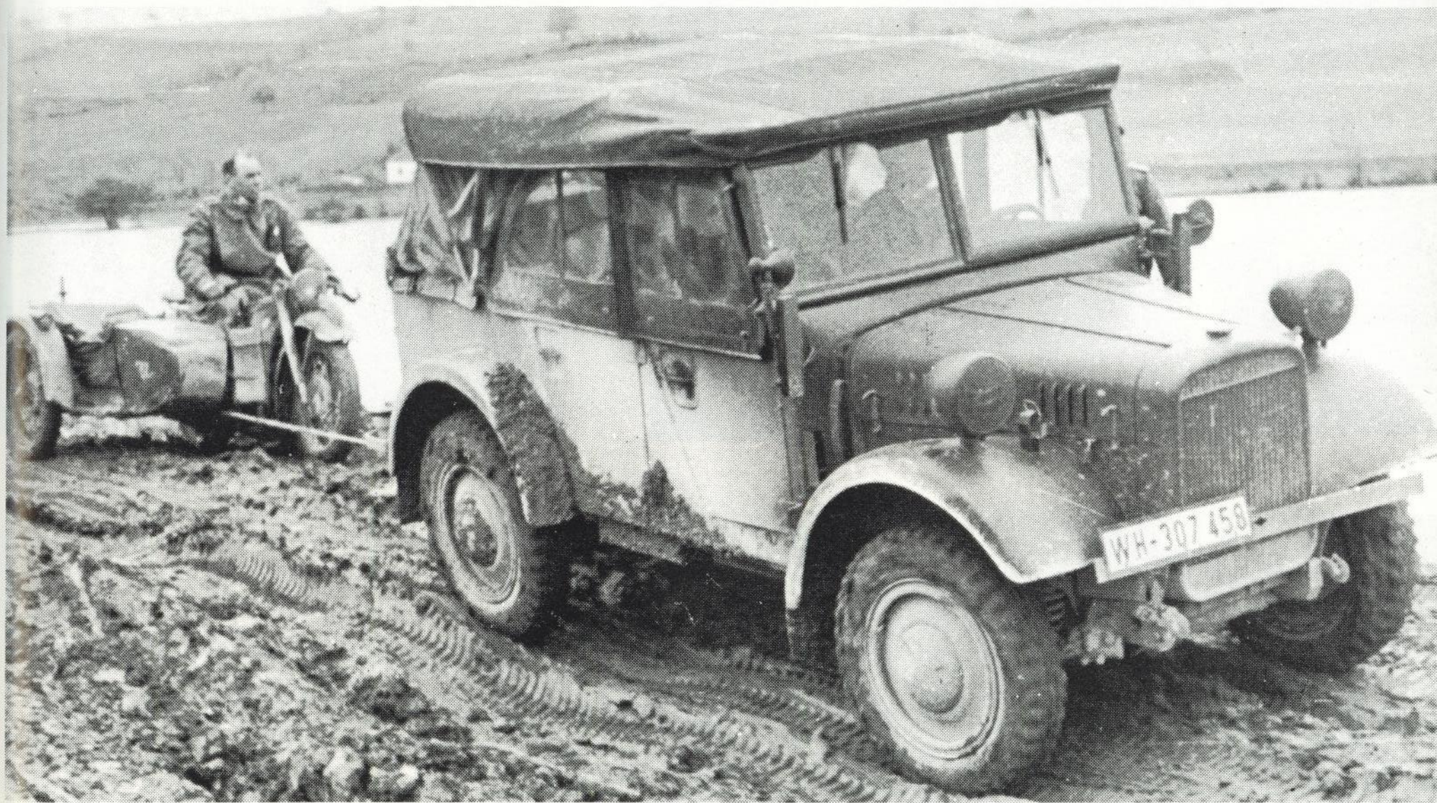
A light uniform personnel vehicle, presumably a "light cross-country-capable personnel vehicle (M. V. 1)", tows a BMW R-75 motorcycle with sidecar. An exact determination of whether this is a "type 40" or an older type of 1st uniform personnel vehicle is not possible on the basis of this photo; only the motor pool sergeant could tell by its papers.
